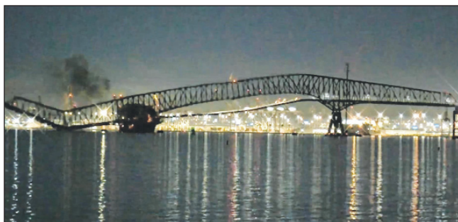
The Francis Scott Key Bridge collapsing.
