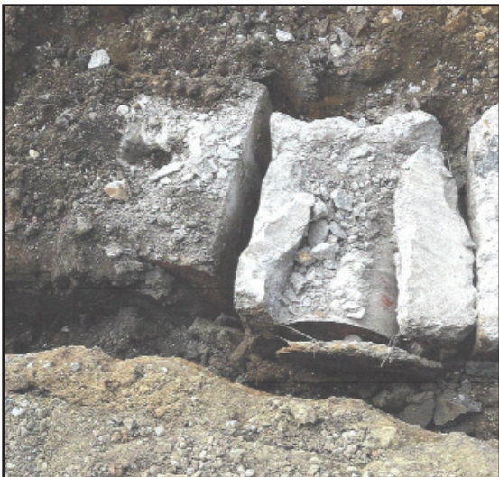
Chemical Waste Drums in Concrete (courtesy TOB)
