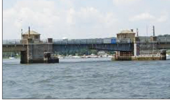
The Bayville Bridge.
