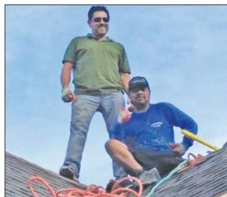
Roofers at Work (Photo courtesy Elite Roofing)
